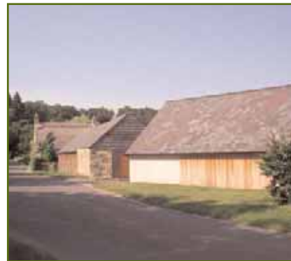
Figure 28 New barns at Wrights Manor
