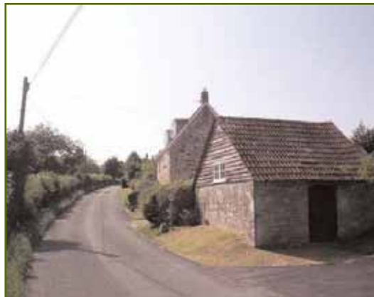
Figure 23 Outbuilding on Snow Hill
