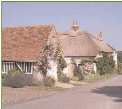
Figure 27 Outbuilding to Cottrells
